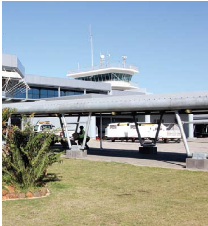
Business continues as usual at East London despite its R180 million runway upgrades
